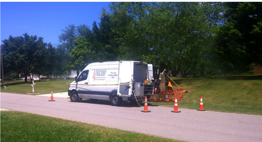
Fig. 1: Underground Cable Assessment.
