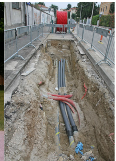
Fig. 2: Wholesale Cable Replacement
