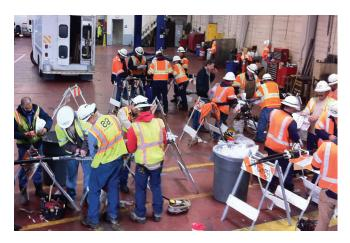
Classroom and field assessments are designed to work together to reinforce accessory manufacturer and utility provided installation training, providing a roadmap for accessory and medium voltage (MV) cable system installation success in four main areas (in order of importance):
