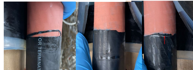
IMPROPER CUTBACKS
